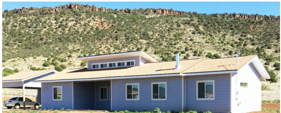
White Mountain Apache Housing Authority (Photo: Travois)
